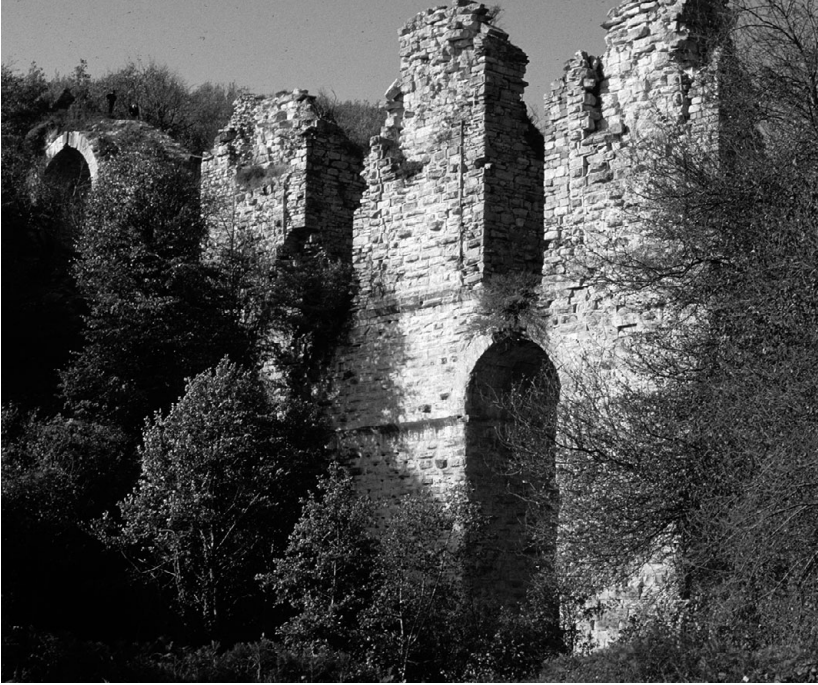
4.3 Büyükgerme aqueduct showing the fifth-century construction similar to Kurşunlugerme and the later narrowing of the upper vaults. (Courtesy of J. Crow)
